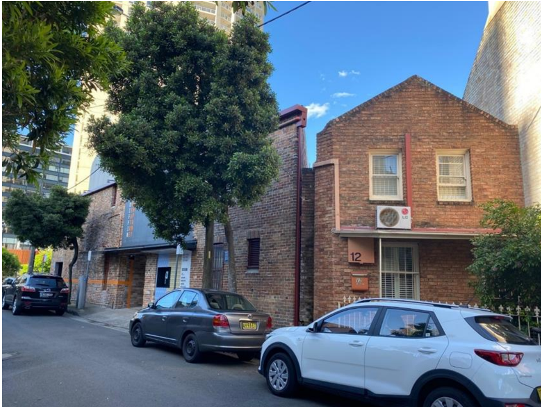
Figure 5: 10 and 12 Nimrod Street viewed from the south-west
