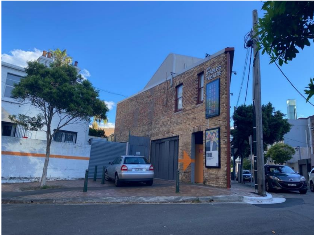
Figure 3: 10 Nimrod Street, viewed from the north-west
